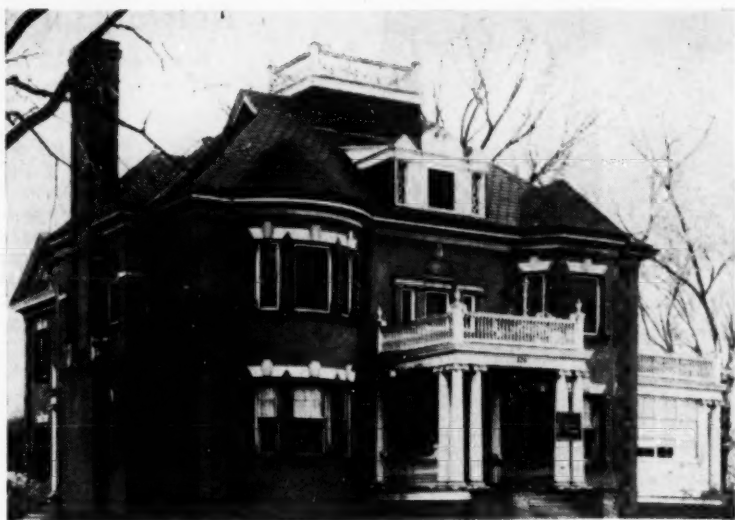
HOME FOR AGENCY MEN —Another agency to get away from the heart of town for its creative efforts is Spitz Advertising Agency, Syracuse, which has taken over this house at 530 Oak St. in Syracuse. The 16-room house, built in 1896, has been remodeled to include a test kitchen, research library and tv film viewing room. The agency's name was changed from William Spitz & Co. with the move.
